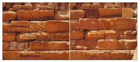
Plate 16. Sample axis at pyramid Beg. N.2 before and after the conservation tests (© RaO, 2016).
