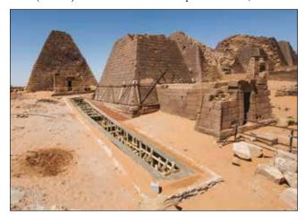
Plate 2. The concrete ring supporting the staircase of Beg. N.9 to prevent a collapse of the stairway walls under the weight of pyramid Beg. N.18, shown during construction in January 2017 (© QMPS, P. Wolf, 2017).
