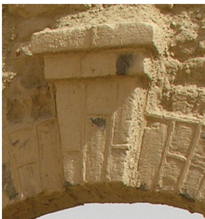
Figure 46. Abu Sillem station, the 'keystone' over the window by the main door.
