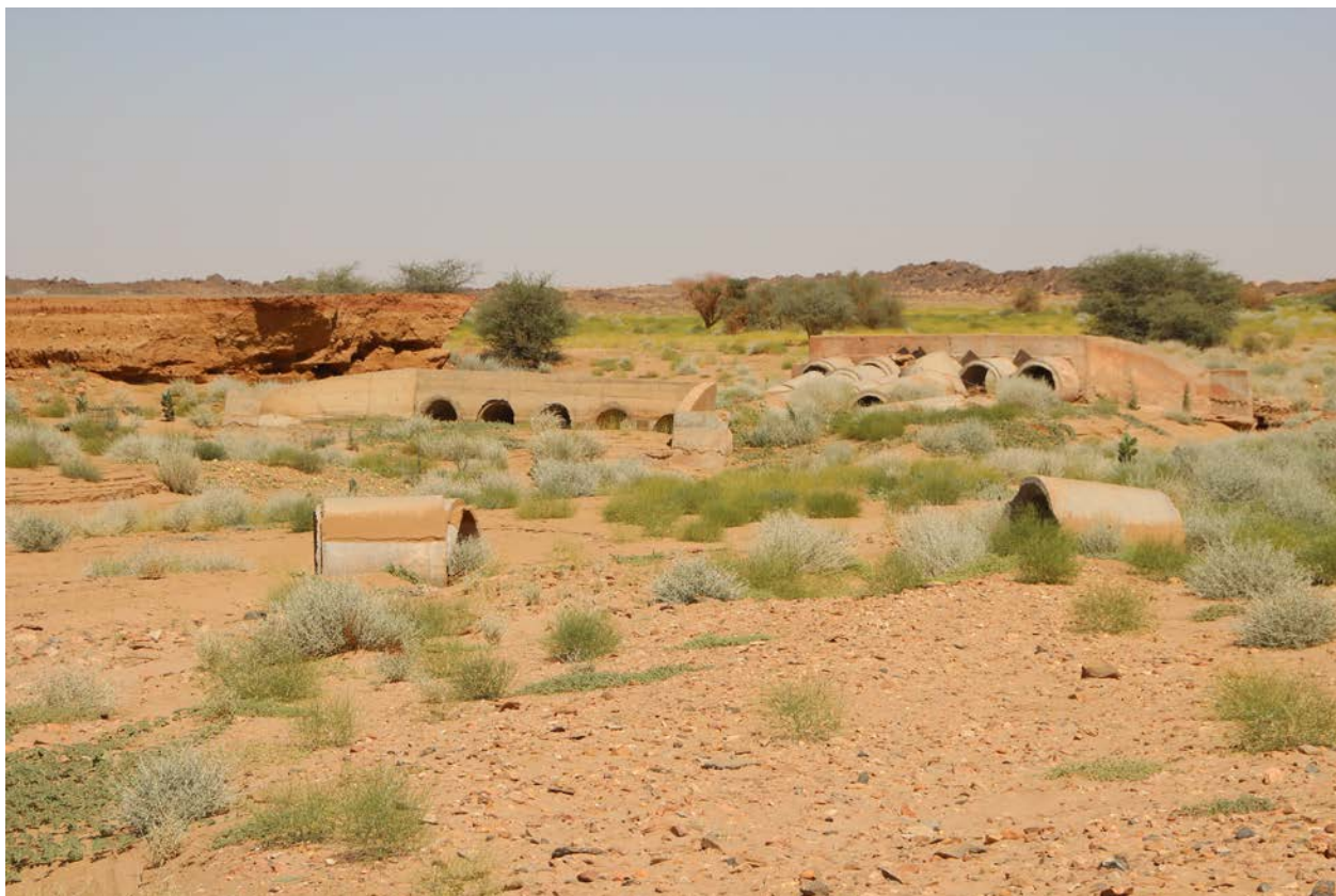
Figure 2. Flood damage to the culverts along the Berber to Abu Hamed road (photo December 2013).
