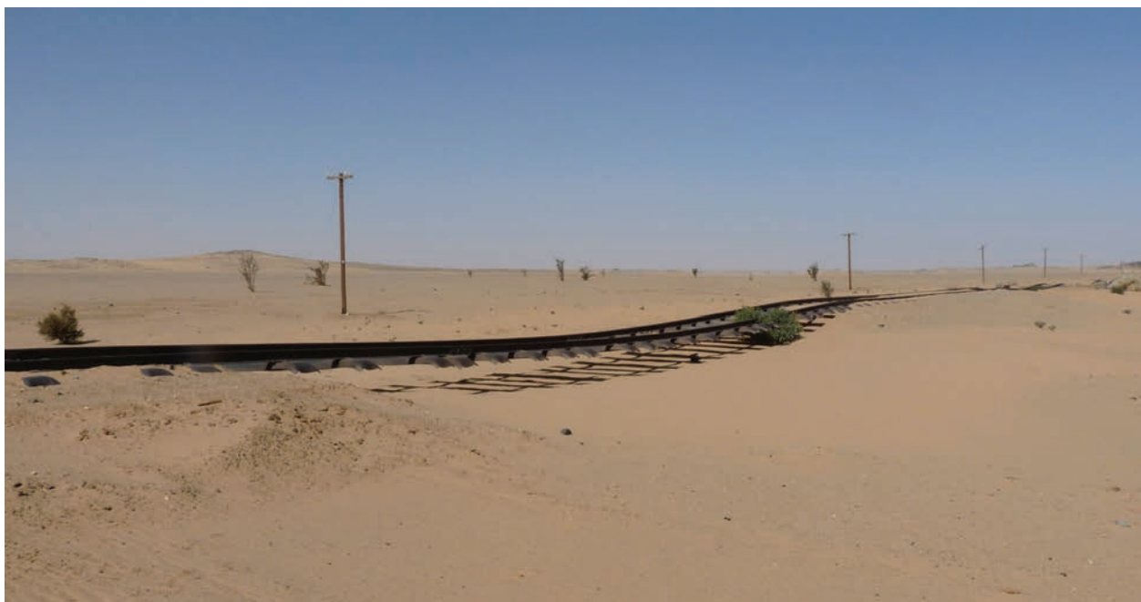
Figure 3. The embankment washed away from beneath a section of the Abu Hamed to Kareima railway line.
