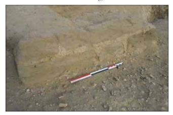
Plate 3. Whitish mortar joining mud bricks.
