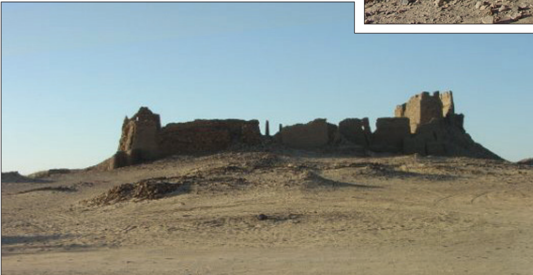
Colour plate XXXVI. Qasr Wad Nimieri. General view of the fort from the north.
