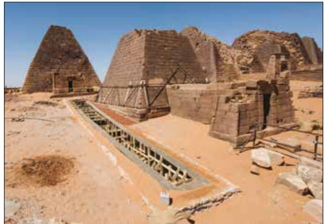
Plate 2. The concrete ring supporting the staircase of Beg. N.9 to prevent a collapse of the stairway walls under the weight of pyramid Beg. N.18, shown during construction in January 2017 (© QMPS, P. Wolf, 2017).
