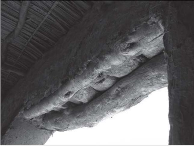
*Plate 12. Umm Quwaib – Detail of logs used for flat lintel.*
