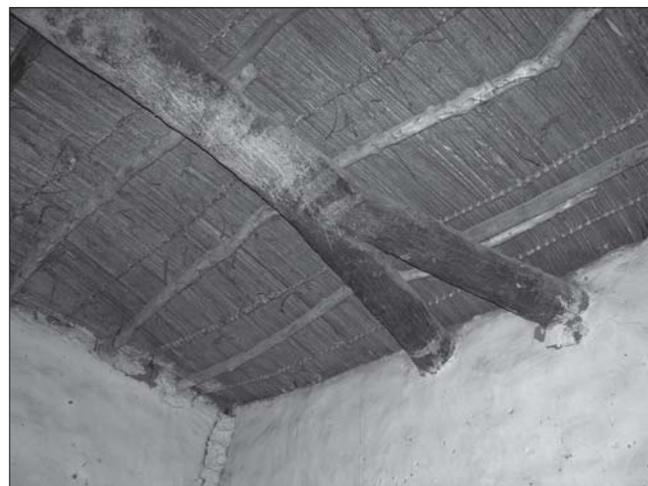
Plate 11. Umm Arosbair on Isheshi Island – the roof structure of room in the diwan.
