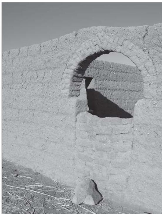
Plate 10. Et-Tereif – stepped arch showing construction of arch from mould-made bricks with block built walls.
