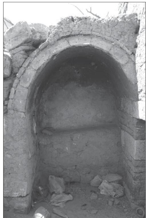
Plate 2. The red-brick barrel vault supporting the stairway in the southern room of House 1.
