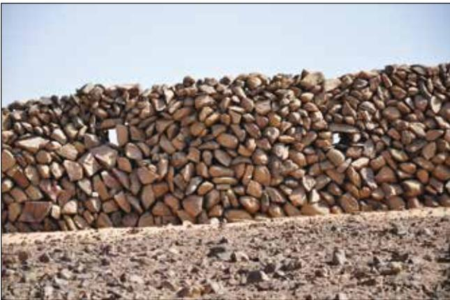
*Plate 4. Section of the perimeter wall at the el-Hisnein-East fort showing windows and inclined stacking of boulders, especially on the left side.*
