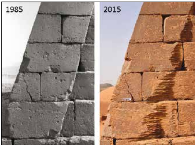
Plate 11. The same pyramid corner in 1985 and 2015 demonstrating the tremendous damage to the monuments due to sand abrasion (left: © DAI, Archive Friedrich W. Hinkel, F-KB-sw-541-21, Friedrich W. Hinkel, 1985; right: © QMPS, Cornelia Kleinitz, 2015).
