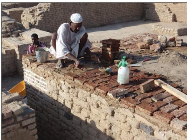
Plate 28. Capping the top of a wall with red bricks
