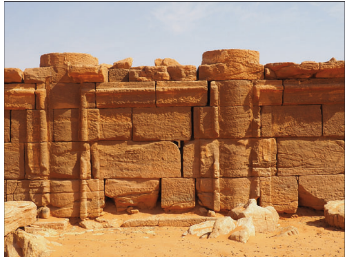
Plate 14. Screen walls of the kiosk walls of the Amun-Temple at Naga.
