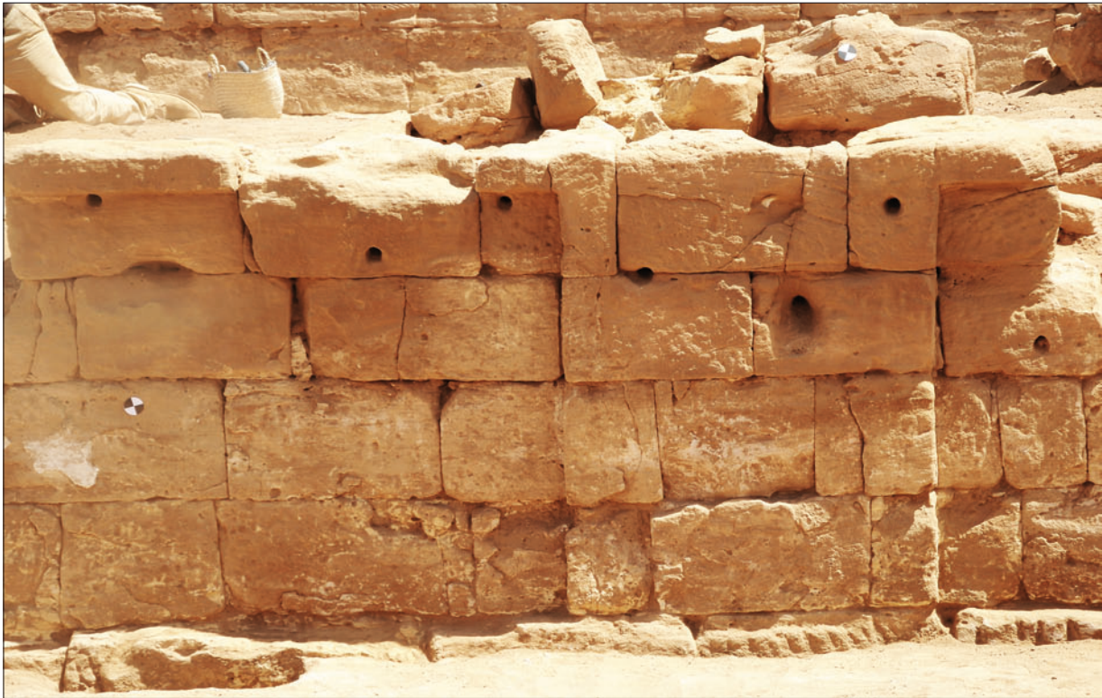
Plate 7. View of the exposed west side of the podium with holes.
