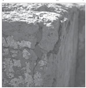
Plate 12. Poor plaster to wall contact.
