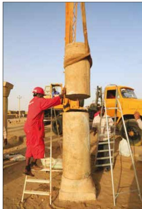
Plate 4. Site DS7, Ganati: positioning the upper part of a broken column shaft into place.
