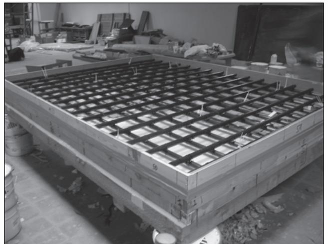
*Plate 14. The grid was laid in the mould.*
