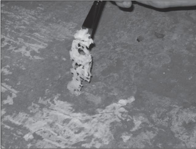
Plate 18. Polyurethane traces are all that was left of the facing.
