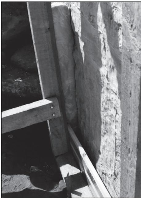
*Plate 5. Shuttering created a space to be filled with polyurethane foam. Note the soft foam wrapped in cling film sealing the gap.*
