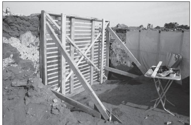
*Plate 7. The frame was cross-braced and timbers were added to rest it on the ground.*
