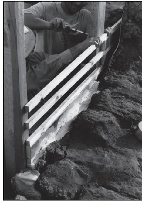
*Plate 6. The shuttering was screwed to the frame.*
