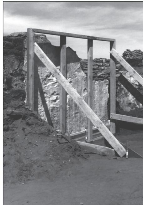
*Plate 4. A frame was set in place and anchored to the ground.*
