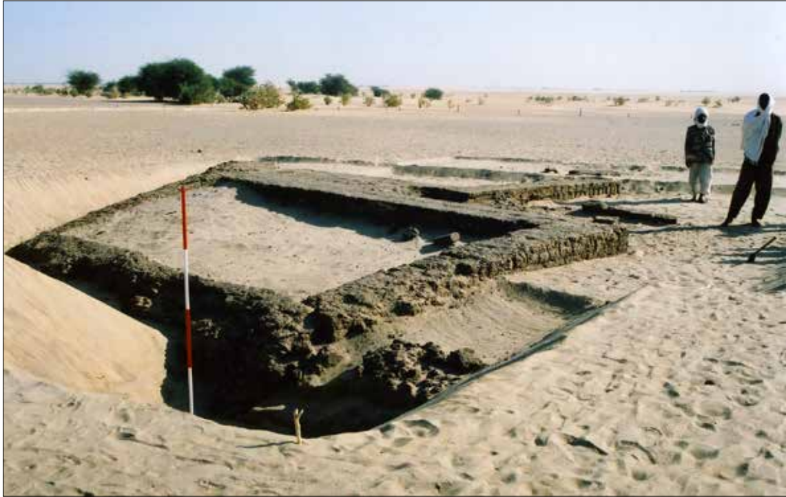
Plate 8.8. General view over Building Z1 during excavation looking north east. The relationship of the denuded walls of room Z1-I to the present ground level can be clearly seen – scale bar 2m.
