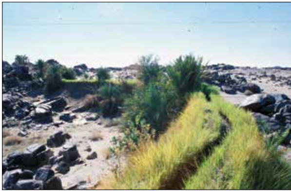
Plate 14. An irrigation channel on a high embankment to supply remote fields in the desert.
