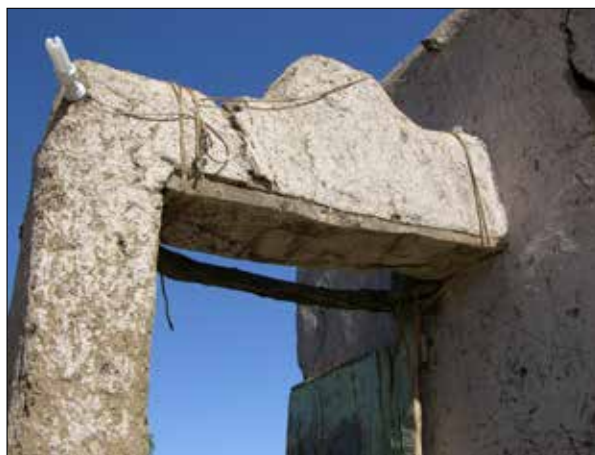
Plate 90. Umm Arosbair, House E1. Detail of entrance doorway with shaped crest of jalous which is supported by a wooden form-board held on by string.
