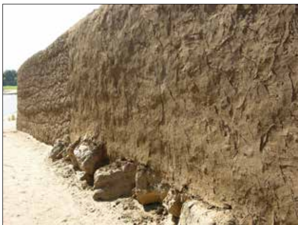
Plate 87. Umm Arosbair. Roughly plastered jalous exterior wall on rocky base.
