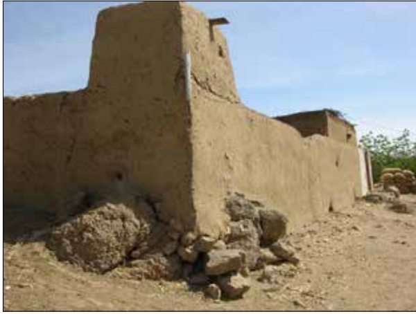
Plate 122. Umm Kedissa, House F2. Exterior view showing pigeon house at corner supported on bedrock foundation.
