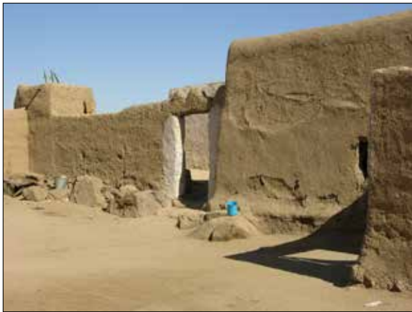
Plate 52. Et-Tereif. Enclosure wall of jalous on boulder foundations – a narrow street.
