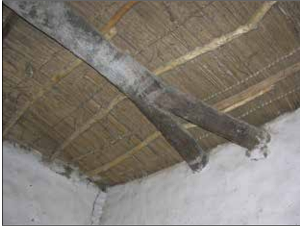
Plate 92. Umm Aroshair, House E1. Ceiling of family room of large log supporting branches and reeds, the ends of the log protruding through the wall as a decorative feature.
