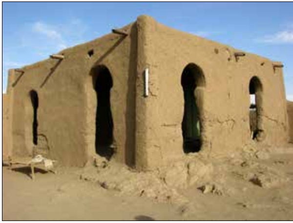
Plate 165. Umm Quweib, House K1. Diwan with keyhole openings in the arcade built on rock foundation.
