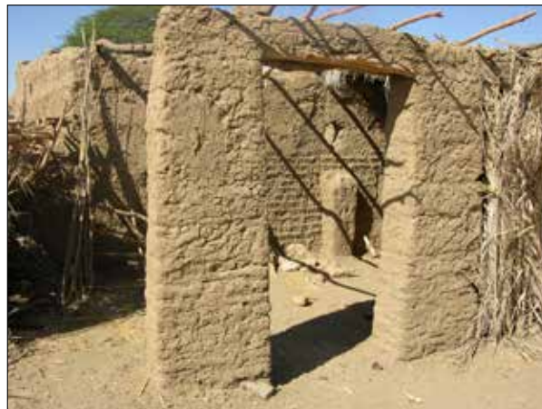
Plate 156. Umm Gemesa. Shaded rakuba of brick columns and palm branches.
