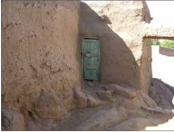
Plate 144. El-Hazama. House walls built on huge protruding rocks with rectangular opening and a door set in corner with doorstep formed from bedrock.
