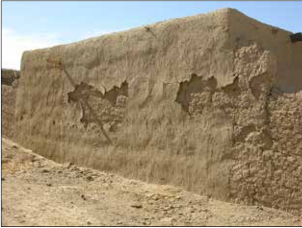
Plate 183. Abu Anghareeb. Jalous enclosure wall with plaster peeling off.
