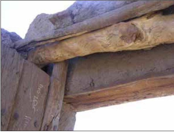
Plate 171. Umm Quweib, House K2. Detail of wooden lintel to entrance door showing pivot socket of wooden door.
