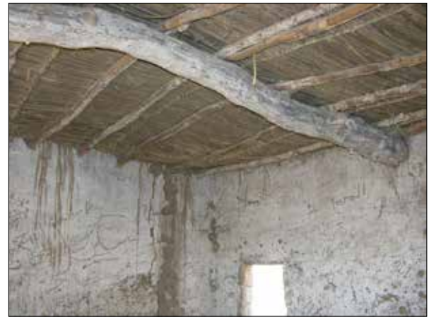
Plate 158. Umm Gemesa. Ceiling of room with plastered walls showing signs of repair at the corner caused by lack of bonding.
