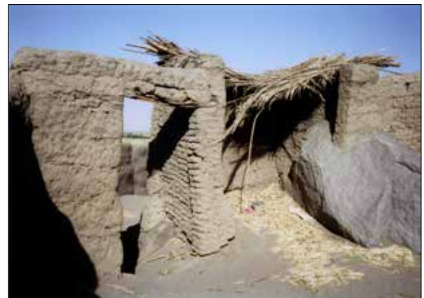
Plate 149. El-Hazama. Walls of jalous and mud brick supported on large boulders and roofed with palm branches
