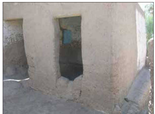
Plate 33. El-Hazama. Rectangular door openings with two-part renewable threshold.
