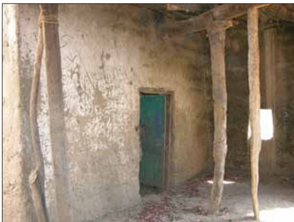
Plate 147. El-Hazama. Interior of house in poor condition showing ceiling beams supported by wooden columns.
