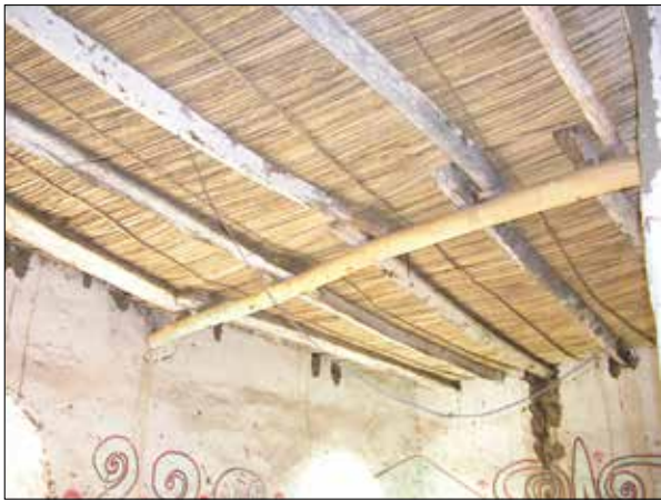
Plate 7. Ceiling of layers of beams and reeds.
