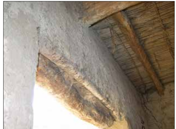
Plate 32. Umm Quweib. Ceiling of palm ribs and lintel of rectangular opening to arcade.
