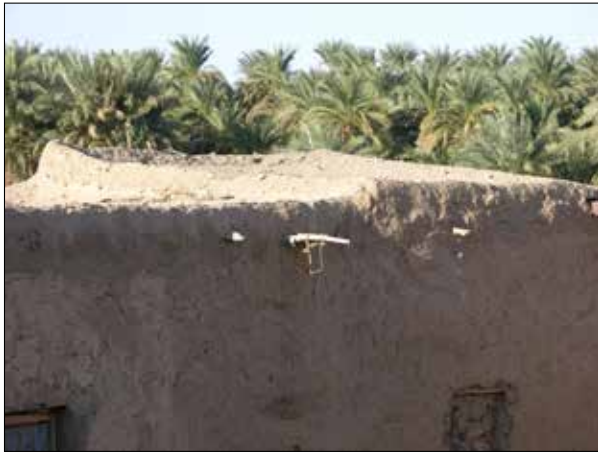
Plate 39. Umm Gemesa. Roof constructed in traditional way with slightly dished plastered surface and water spouts for drainage.
