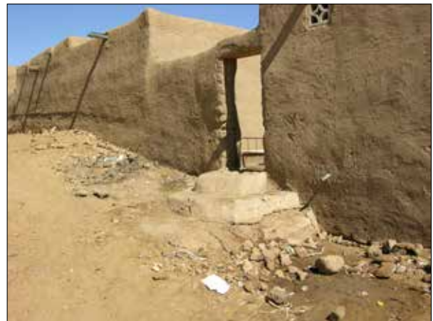
Plate 120. Umm Kedissa, House F1. Exterior wall showing steps leading up to kitchen entrance back door and showing wall construction rising up according to ground level.
