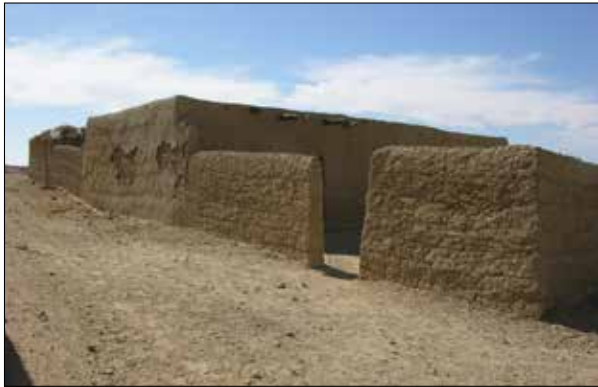
Plate 20. Abu Anghareeb. Jalous enclosure wall of courtyard, house and rear yard built on a slope.
