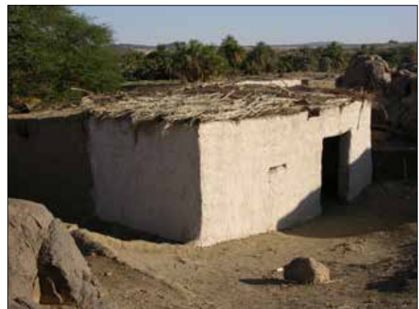
Plate 38. Umm Gemesa. Roof strewn with palm fronds and reeds.
