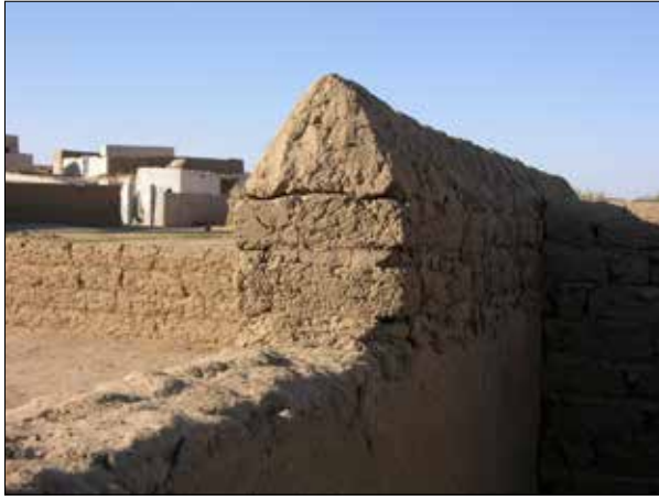
Plate 18. Et-Tereif. Triangular-shaped coping on the enclosure wall of the mosque.
