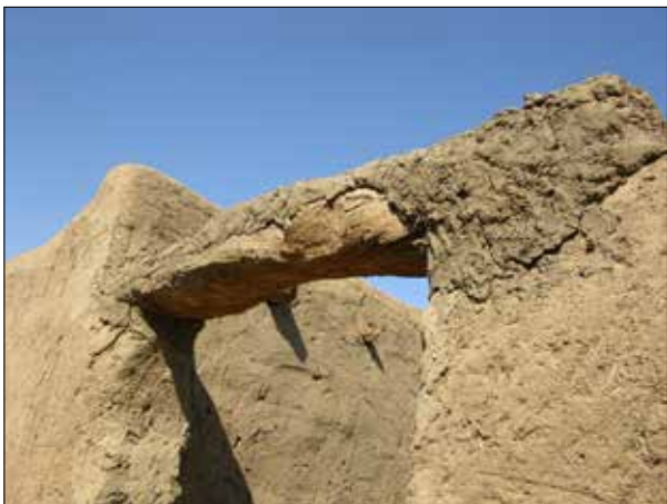
Plate 167. Umm Quweib, House K1. Doorway to the family house showing wear of mud plaster on lintel revealing the wood beneath.
