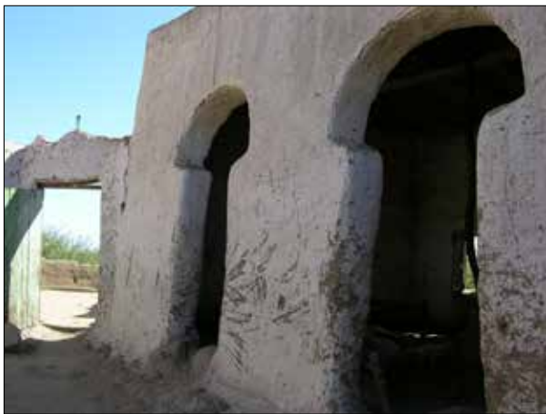
Plate 93. Umm Aroshair, House E1. Exterior wall of family room facing courtyard with arcade of keyhole openings and doorway to diwan.
