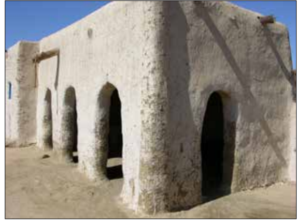
Plate 63. Et-Tereif, House A2. Summer berandah with rounded arches and buttresses at corner – all plastered white.
