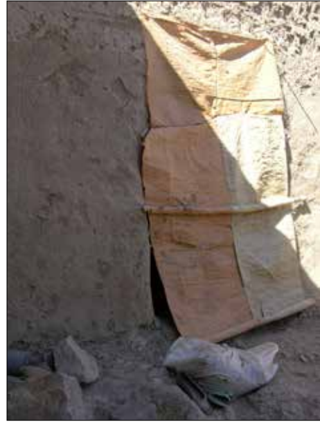
Plate 174. Umm Quweib, House K2. 'Mat' of paper sacks released to keep sand and heat out of living area.
