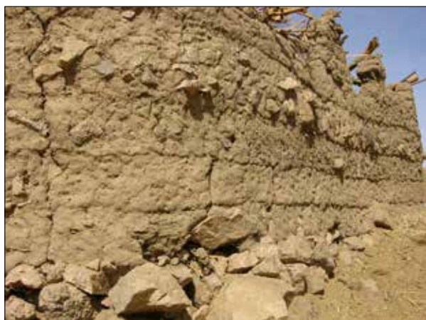
Plate 11. Umm Kedissa. Unplastered enclosure wall of jalous on a foundation of various sized boulders.
