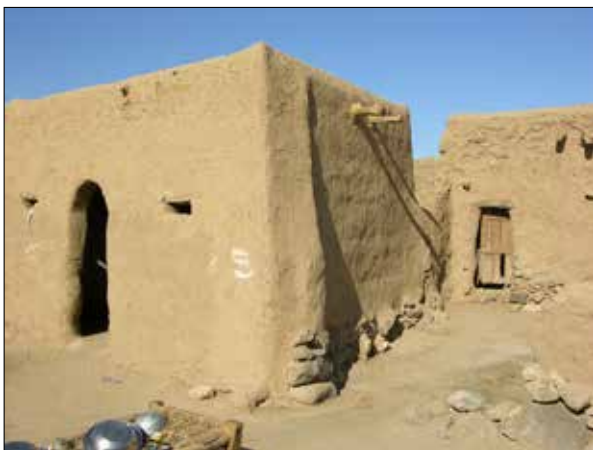
Plate 86. Hantilah. The father's house with rounded openings, corner buttress and two rain spouts.
