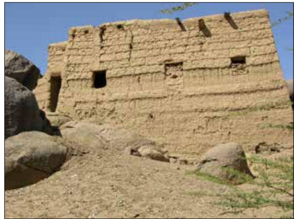
Plate 141. El-Hazama. Wall of deteriorating jalous built on uneven rocky foundation.
