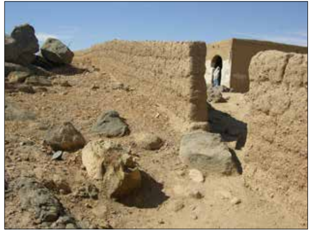
Plate 187. Abu Anghareeb. Enclosure wall of jalous which reduces in height to accommodate the sloping ground, with boulder used for threshold of doorway into the courtyard with house.
