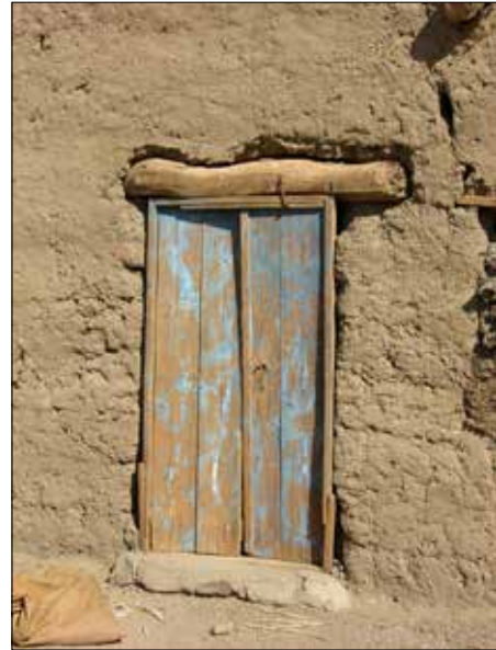
Plate 31. Mis Island. House door with a large exposed timber lintel, two-leafed wooden door and doorstep.
