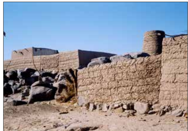
Plate 5. Abu Angareeb. House wall of sections of jalous built on top of protruding bedrock with mud-brick repair.
