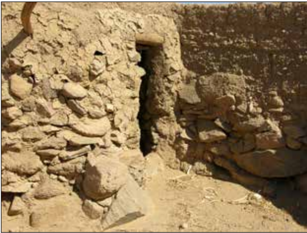
Plate 6. House walls of stones embedded in rough jalous built on loose boulders and protruding bedrock.
