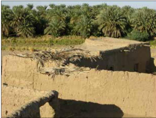
Plate 155. Umm Gemesa. Plastered and dished roofs to the houses.
