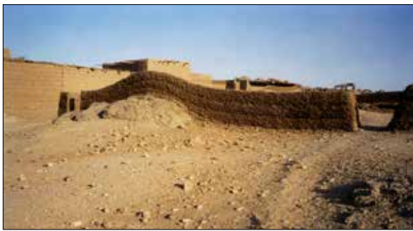
Plate 19. North of Et-Tereif. Wall of jalous laid on undulating ground to create a "wavy" wall.
