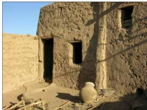
Plate 28. Umm Gemesa. Exterior of a house with door and window openings and details of a buttress and low mastaba.
