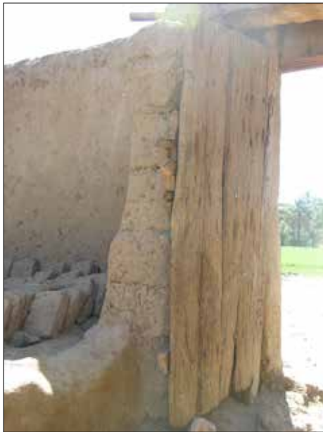
Plate 35. Umm Quweib, Building K2. Main entrance door of traditional wooden form, opening inwards to the courtyard.
