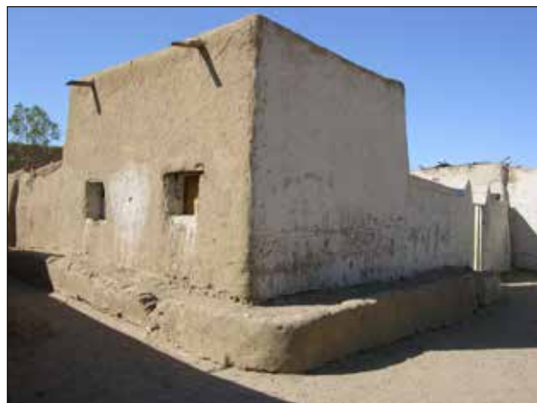
Plate 135. Umm Kedissa, House 5 'mastaba house' enclosure wall including two sides of a room and the main entrance facing the plaza. A mastaba is built around the base of the walls of the room.
