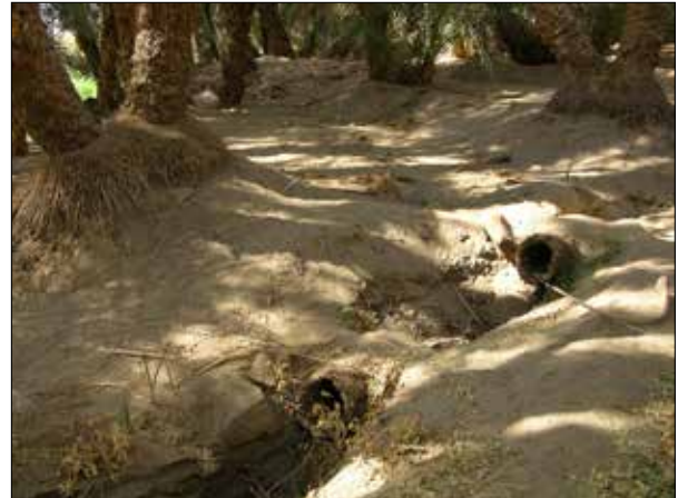
Plate 223. Hollowed palm logs making water pipes for irrigation in palm groves.
