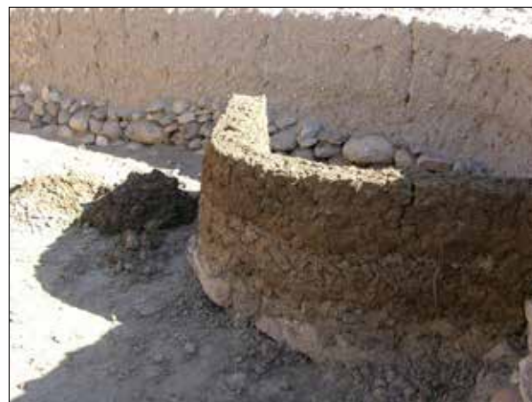
Plate 12. Hantilah. Unfinished semi-circular animal pen showing jalous construction in progress: heap of prepared mud and stone mixture beside two stages of wall.
