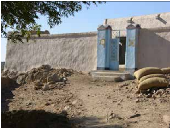
Plate 139. Umm Kedissa, House F6. Well-built plastered and painted white enclosure wall with imposing entrance gateway of rectangular painted posts flanking two-leaf metal door.
