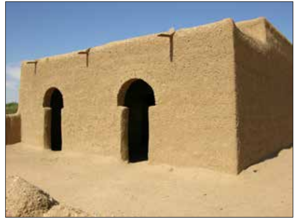
Plate 74. Et-Tereif, House A5. Newly built house with two keyhole openings and showing two levels of roofing.
