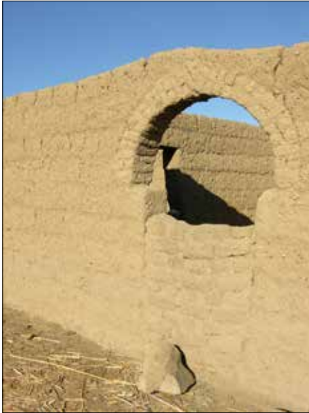
Plate 14. Et-Tereif. Conventional arched opening made of mud bricks inserted into a jalous wall.
