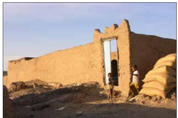
Plate 100. Umm Kedissa. Enclosure wall of house with shaped crest over entrance door and protruding rocks in roadway some used as wall foundations.
