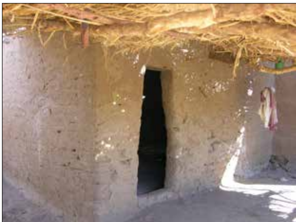
Plate 40. Umm Quweib. Area outside kitchen shaded by palm fronds resting on beams.
