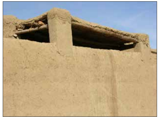
Plate 106. Umm Kedissa. Outer enclosure wall supporting columns for interior loggia.
