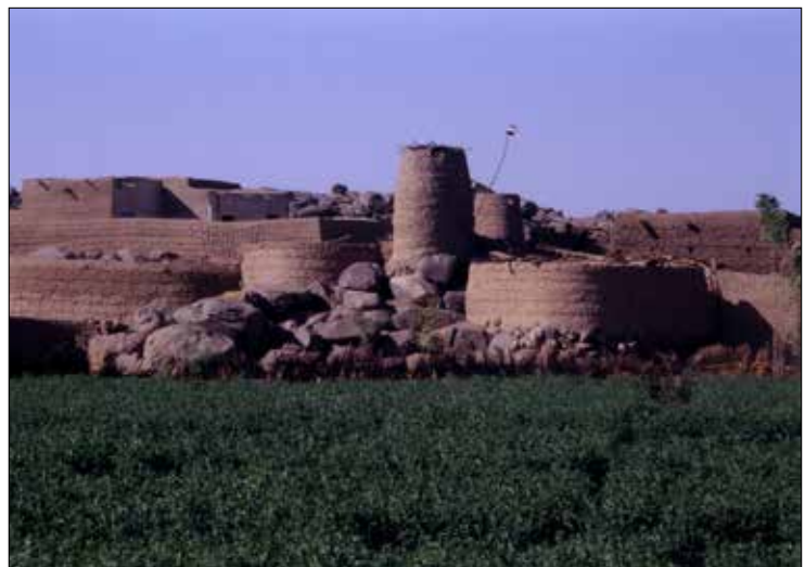
Plate 75. View of Ganob from the surrounding fields showing jalous walls, both horizontal and circular, and circular pigeon loft, all built on a foundation of boulders and bedrock.
