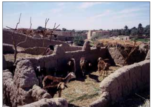
Plate 224. Abu Anghareeb. Animal pen of jalous on rock foundation.
