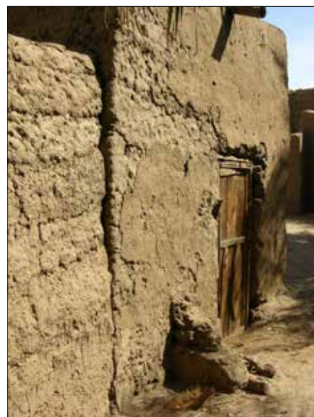
Plate 142. El-Hazama. Walls in the village of deteriorating jalous, showing lack of bonding and poor state of the door.
