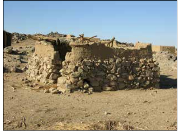
Plate 84. Hantilah. Animal pen of stone wall topped with jalous .
