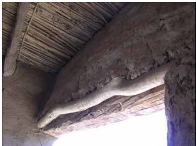
Plate 176. Umm Quweib, House K3. Exposed wood of lintel of rectangular opening.
