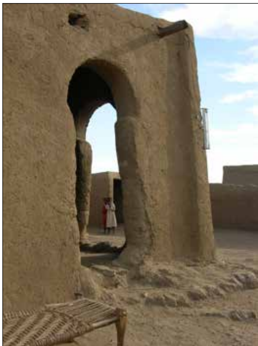
Plate 166. Umm Quweib, House K1. Corner of diwan arcade strengthened by a buttress.
