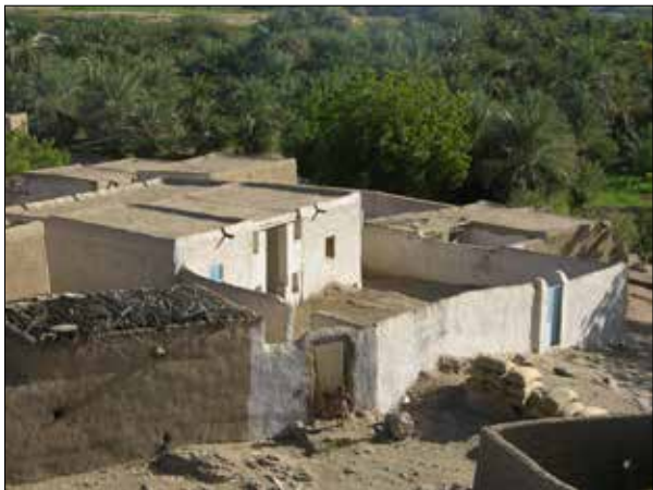
Plate 124. Umm Kedissa, House F2. The diwan with entry gap broken through party wall. A well plastered house with rectangular openings and plastered enclosure wall.
