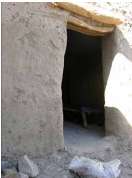
Plate 173. Umm Quweib, House K2. Rectangular opening to arcade with rolled up 'mat' of paper sacks above lintel.
