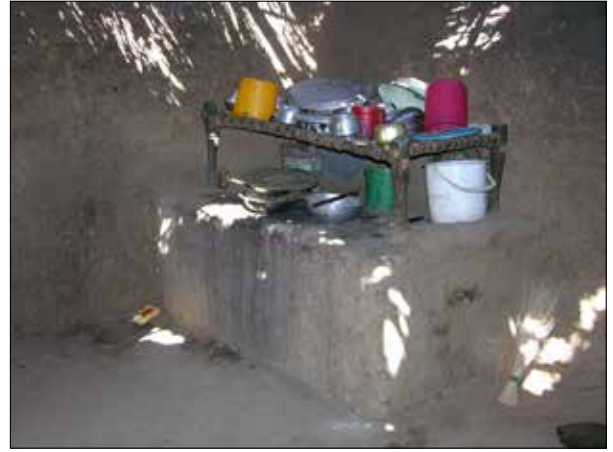
Plate 180. Umm Quweib. Kitchen where protruding rocks have been used as a base to support cooking equipment.
