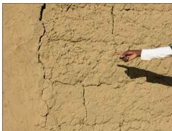
Plate 13. Et-Tereif. Finished section of jalous wall showing size of marked "bricks" (adult hand for scale).
