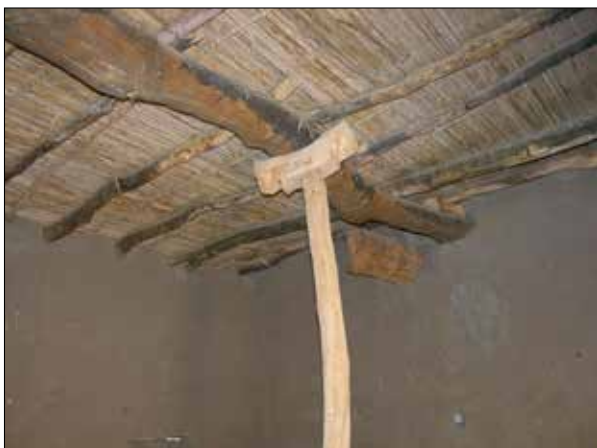
Plate 157. Umm Gemesa. Ceiling with supporting wooden posts.
