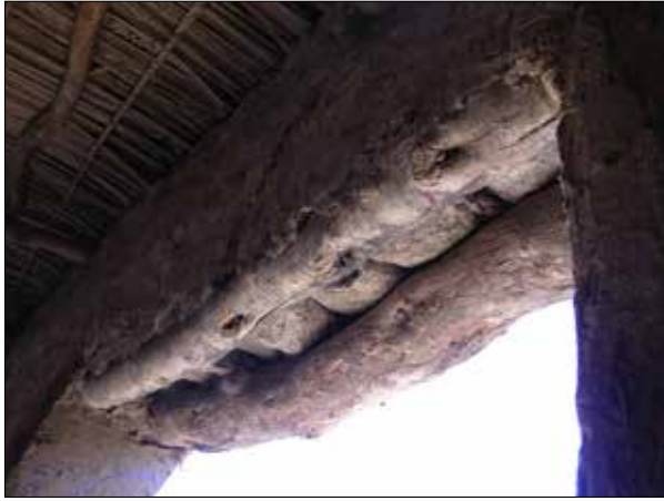
Plate 177. Umm Quweib, House K3. Exposed wood of lintel of rectangular opening.
