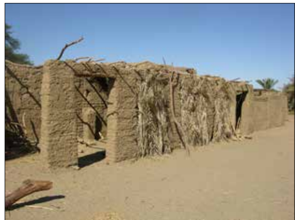
Plate 27. Umm Gemesa. Shelter in courtyard of brick pillars roofed with palm branches.
