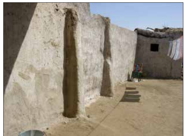
Plate 57. Et-Tereif, House A1. Buttress supports to plastered interior wall of second courtyard, with kitchen building at rear.
