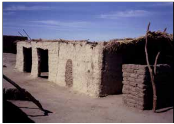
Plate 198. Abu Anghareeb. House with rectangular arcade openings with kitchen attached having a round-arched opening filled with mud brick and a shaded rakuba and zir place.
