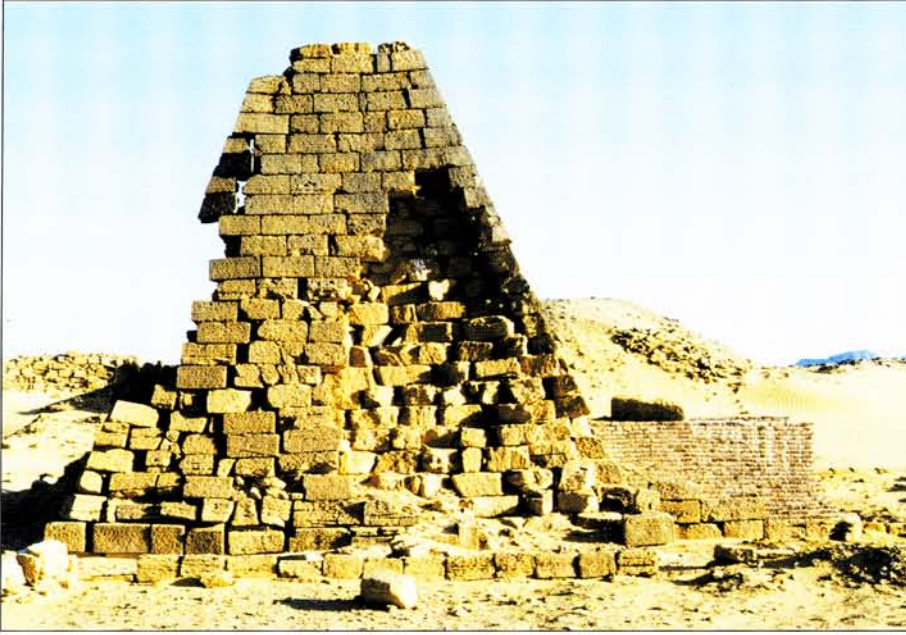
Plate XIII. Meroe. Pyramid BEG W 18: Structural situation in December 1997 after the beginning of the restoration of the offering chapel. (Ph. 430/32).
