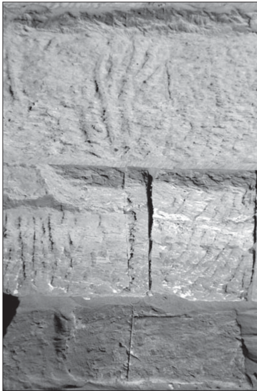
Plate 3. Centre line of a pyramid engraved on the projecting foundation block and on the first stone course as a line. From the second course onwards the centre line continues as an engraved mark on the edge of the stone. (slide 9761)
