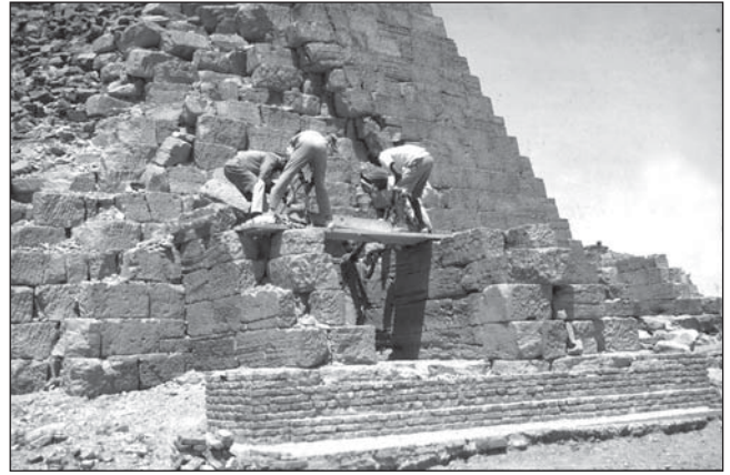
Plate 7. Chapel of pyramid BEG S 5: Beginning of work on the foundation and roofing. (slide 10924)
