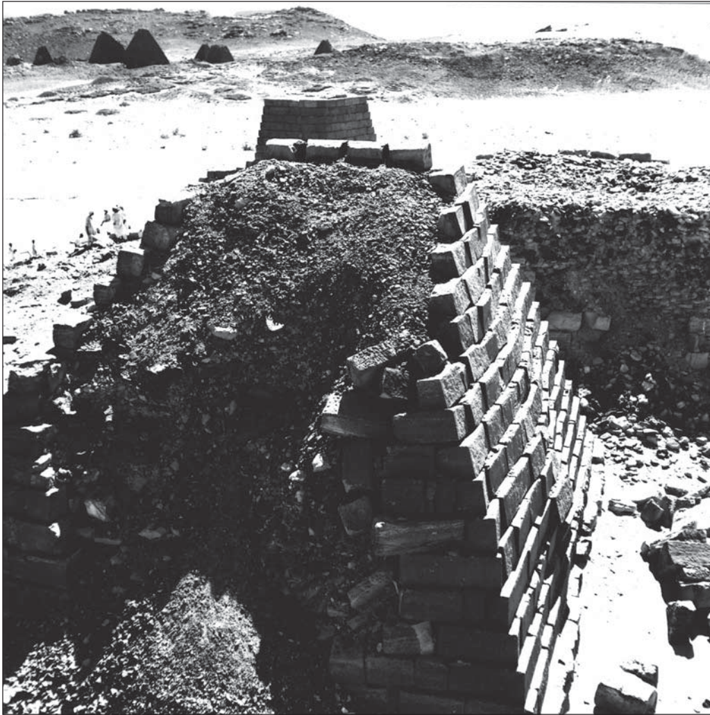
Plate 1. Pyramid BEG N 3: Internal filling encased with only one row of mantle stones. (Ph. No. R 537/3)
