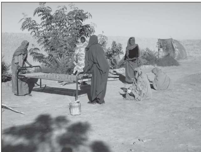
Plate 15. Laying out the structure's plan using a bed as the unit of measure.
