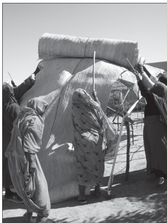
Plate 19. Installing the mat roofing.
