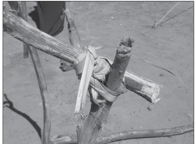
Plate 17. Pliable palm fronds used to secure the roof beams.
