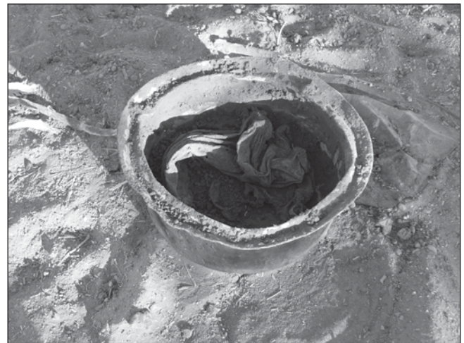
Plate 13. Mixture of crushed red brick and gum arabic used to treat the wooden beams.
