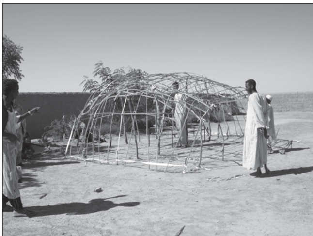
Plate 18. Completed wooden skeletal framework.
