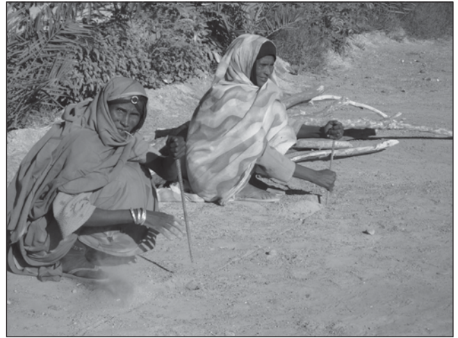
Plate 16. Digging holes for posts following an outline drawn on the ground.
