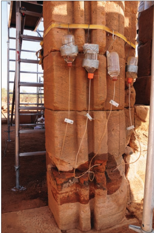
Plate 25. Lower courses of stones in the Hathor Chapel on drips with conservation fluid applied over many days.
