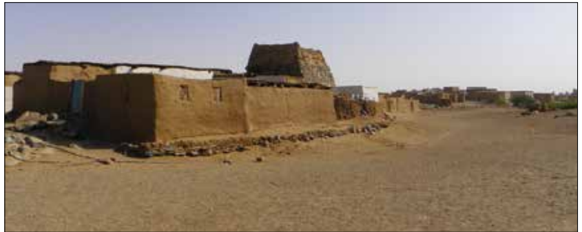
Plate 9. The western diffi is part of a modern dwelling (photo A. Misiurny).
