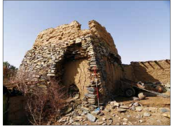
Plate 8. Western diffi. It was built from stone and mud brick; after heavy damage, renovated using jalous technique (photo A. Misiurny).
