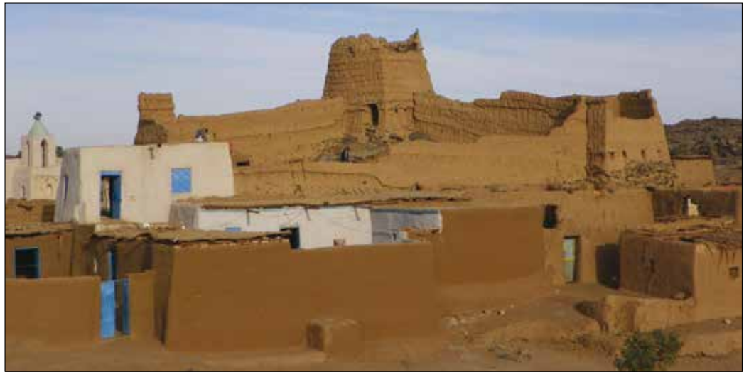
Plate 3. Eastern diffi, mosque's minaret visible on the left side; white plastered building attached to fortifications is now adapted as a room for a married couple (photo. M. Drzewiecki).
