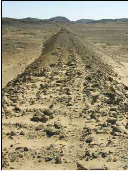
Plate 24. Locus 25. Well preserved rail bed with position of sleepers visible.
