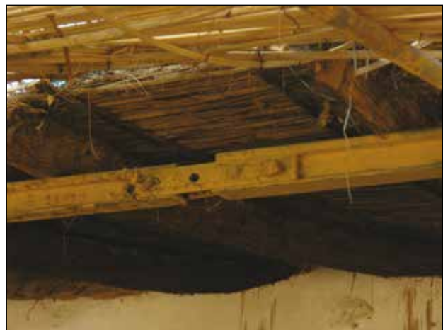
Plate 40. Rails with fishplates supporting a roof in the souk at Delgo.
