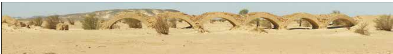
Plate 56. Locus 197. The eight-arched stone, red brick and concrete bridge.
