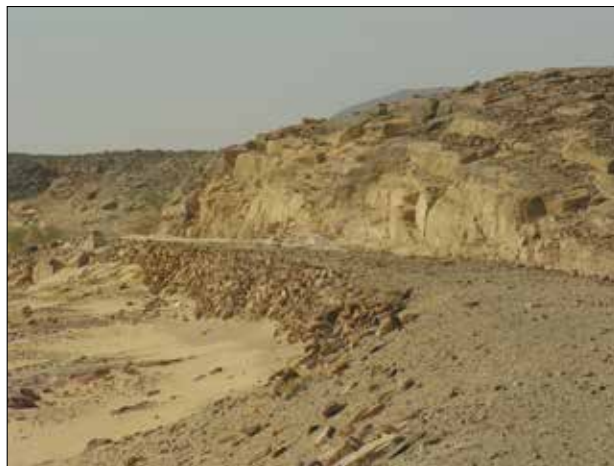
Plate 49. Locus 230. Cutting and embankment on the second phase line by the bridge at Kajbar.
